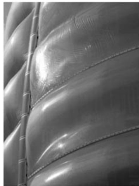
Fig. 1. The ETFE pneumatic double-membrane "pillows" of the façade of the Space and Science Center in Leicester, UK. ETFE, a member of the fluoroplastic family, offers excellent transparency, good mechanical strength, good permeability resistance, and excellent abrasion resistance over a temperature range of -185^{\circ}\text{C} to +150^{\circ}\text{C} . [Photo by J. E. Fernández]
